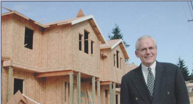
During construction of the duplexes.
