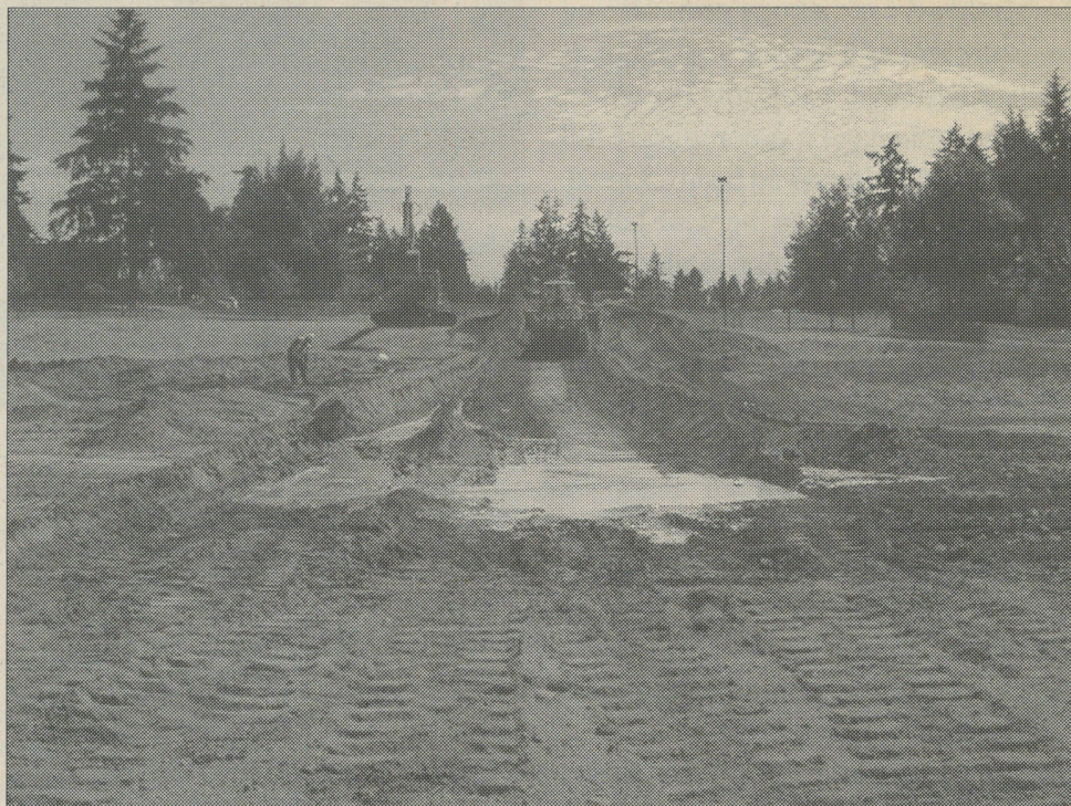
Construction workers remove topsoil from The Green during preliminary digging.
