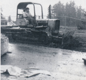
Preparation for foundation of new married students' apartments
