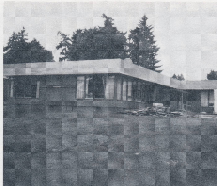
Construction is well underway on the Student Union Building exterior renovation.
