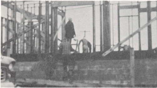
Students "in action" on construction of the chapel.
