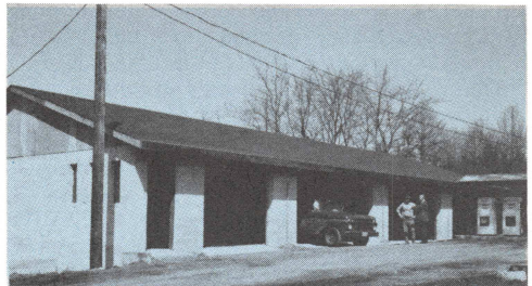
Owen Hodges and Martin Dormier in front of new maintenance and bus garage.
