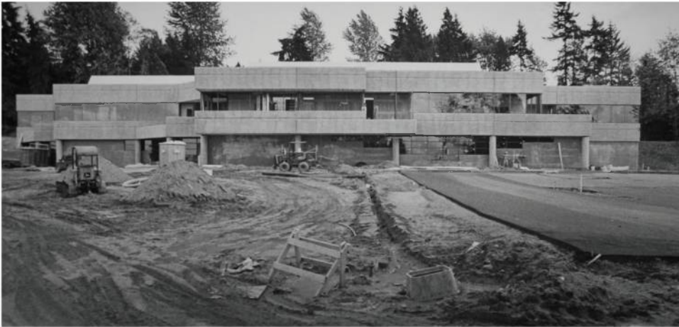
The Seahawks headquarters under construction.
