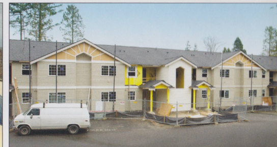
NEW APARTMENTS – Nearing Completion
