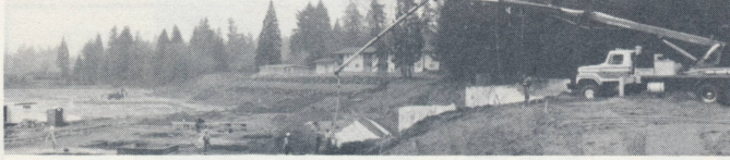
Footings of Administration and Training Facilities are poured while fields are leveled.
