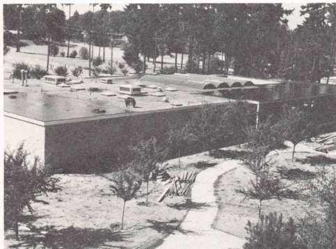
Exterior view of cafeteria
