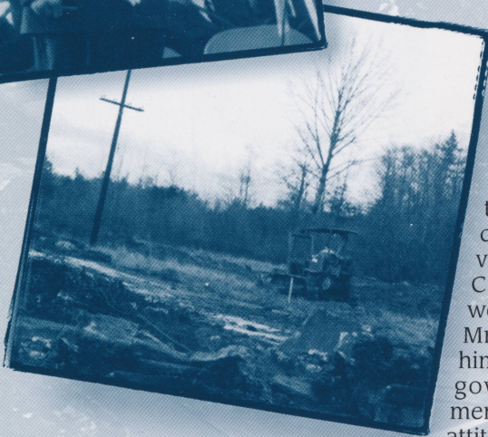
Top: President Butterfield speaking at the Northwest College ground-breaking ceremony. Bottom: Clearing the way for a brighter future.
