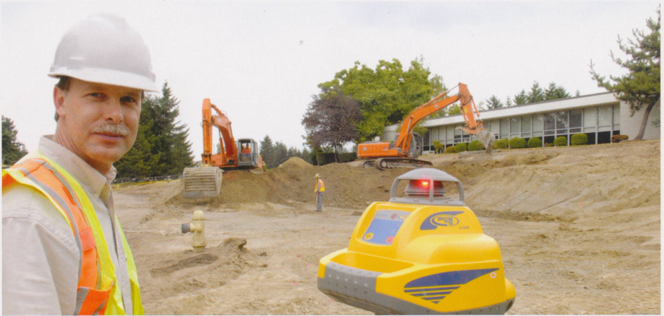
Steve Sankey, Director, Campus Planning and Construction, next to a laser level used to establish the bottom level of the new Health and Sciences Center at Northwest University.
