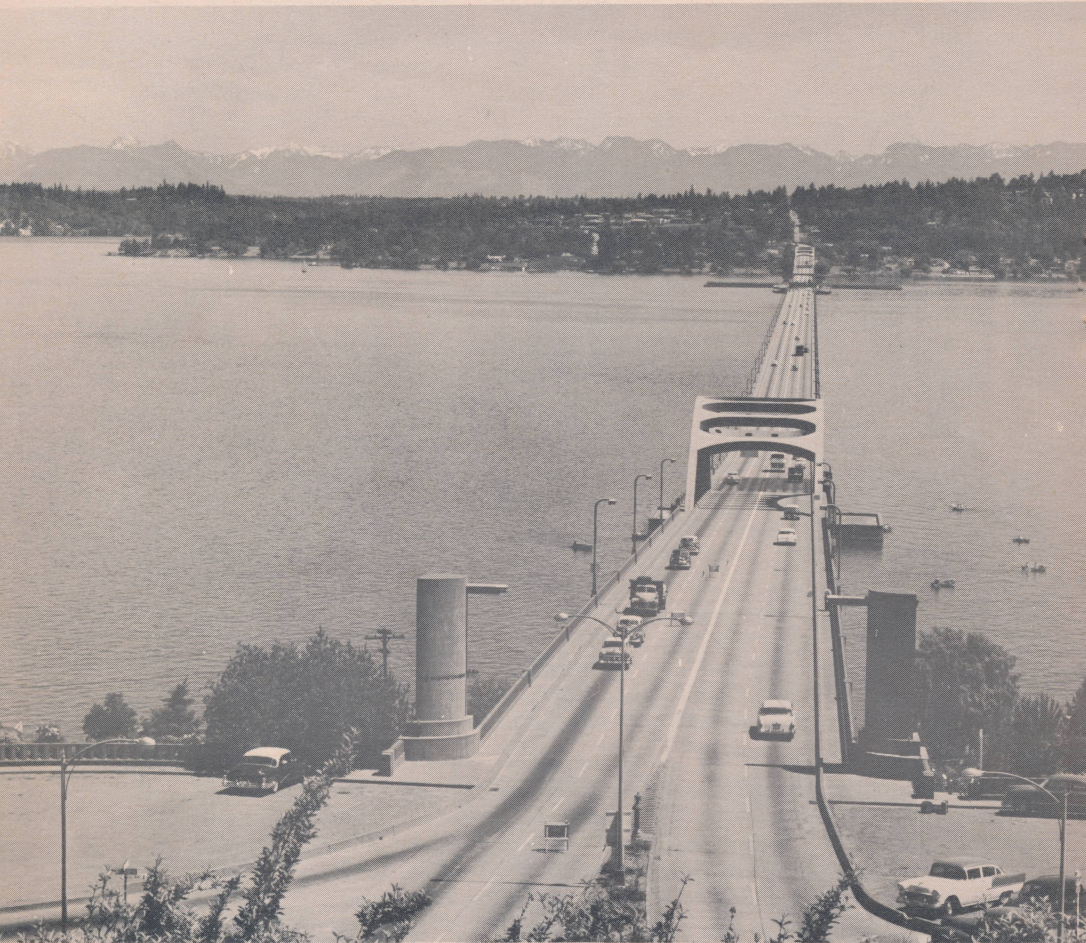
Lake Washington Floating Bridge
