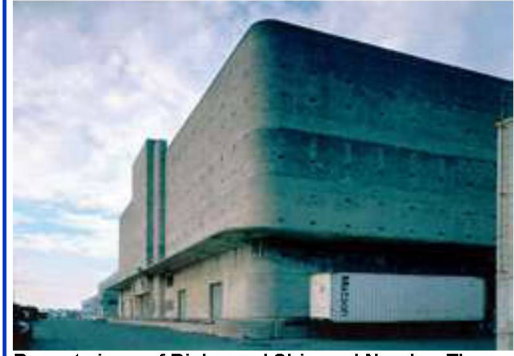
Recent views of Richmond Shipyard Number Three including two warehouses and cranes Photos courtesy of Lisa Pfueller Davidson and from the HAER collection (General warehouse view by Jet Lowe, HAER no. CA-326-B-7)
