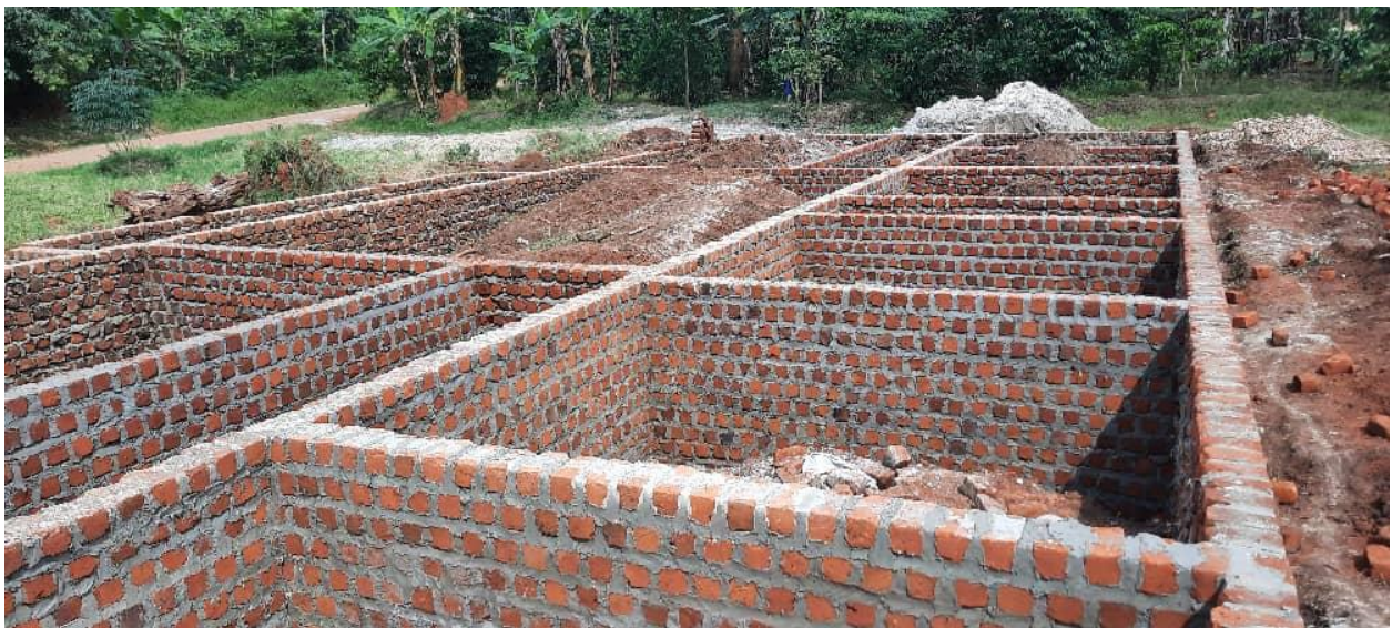
Picture 1: The foundation of Grace Medical Center.
